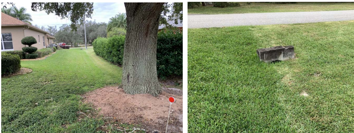
Culvert crossing and side lot ditch taking water towards the Golf Course
