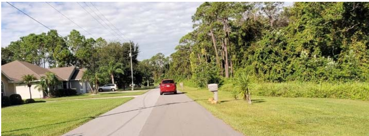
Dog Leg Dr. – Very little ditch present on either side of the road.
